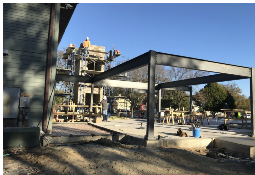
Our future reception and elevator shaft begin to take shape
